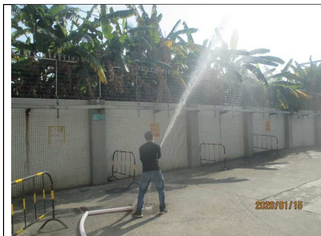
Fire hydrant testing
